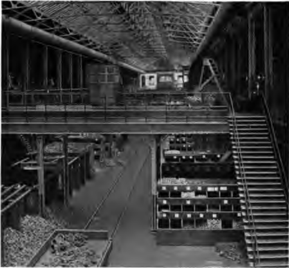
Central Aisle of Machine Shop
